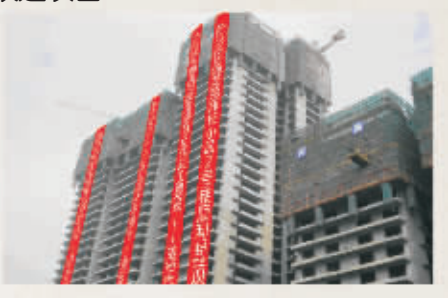
涪龙苑商住小区2#楼顺利封顶
